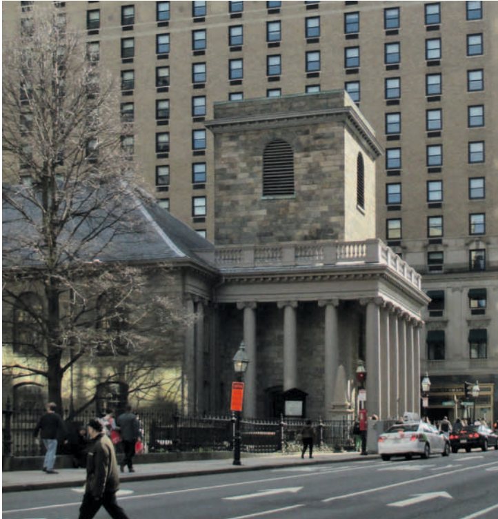
Fig. 3. The tower and portico from Cambridge Street. ( Aaron Helfand )
